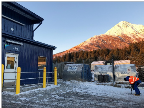
Exhibit 2-1: Field staff use a rotary drill to sample the asphalt profile outside the Alaska Air Cargo building at the ADQ.
